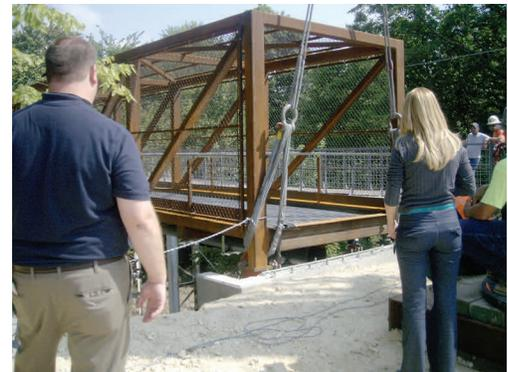
In May 2007, the City of Warrenton was notified by the Norfolk Southern Railroad that the pedestrian bridge which crosses the tracks on Steinhagen Road was failing and needed to be removed. Inspections had shown substantial failures in the foundation and bridge substructure.
