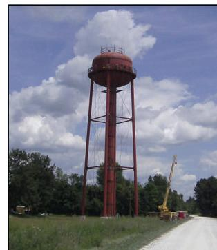
Work is progressing on the City of Hawk Point's water improvement project. A new 100,000 gallon elevated water storage tank has been constructed which will enable the city to meet the daily demands of the community without having water shortages. It will also enable the city to meet Missouri Department of Natural Resources regulations. The photos above show the progression as work is being done on the tower which still needs to be painted inside and out.
